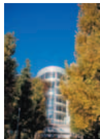
Sousoukan Building on Yagami Campus
